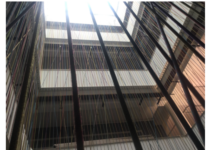
Work in progress in Utrecht.
